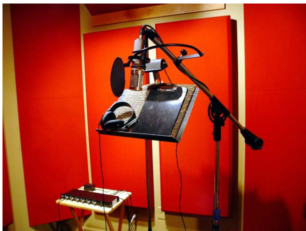
Auralex ProPanels and CT45 Bass Traps in a studio in Nashville, TN. Try varying the distance between you and a boundary, and alternating which direction you face. The differences in tonal character can be pronounced. Notice how the ProPanels are stood off the wall, which increases their absorption & looks great.
