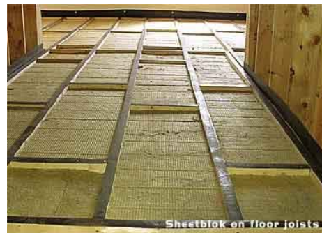
SheetBlok on floor joists
