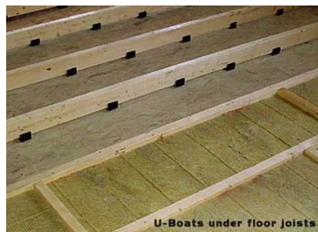
U-Boats under floor joists
